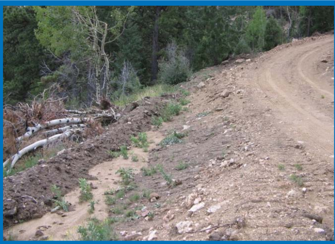
Managing road runoff begins during construction by using dirt berms and brush barriers, which are more effective than a silt fence.
