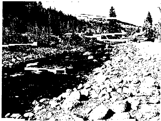
Facing Downstream from the Right Bank
