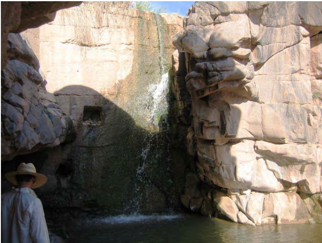
Reach 1 Diversion Barrier
