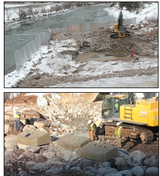
Figure 9. Construction of the Glenwood Springs Whitewater Park during the winter of 2007-2008. In the top photo, a coffer dam diverts the flow of the Colorado River as work is completed on the drained riverbed. In the lower photo, construction crews install wave-generating features, which could qualify as “physical control structures” for purposes of a petition for a RICD water right by the City of Glenwood Springs. (Glenwood Springs Whitewater Park)
