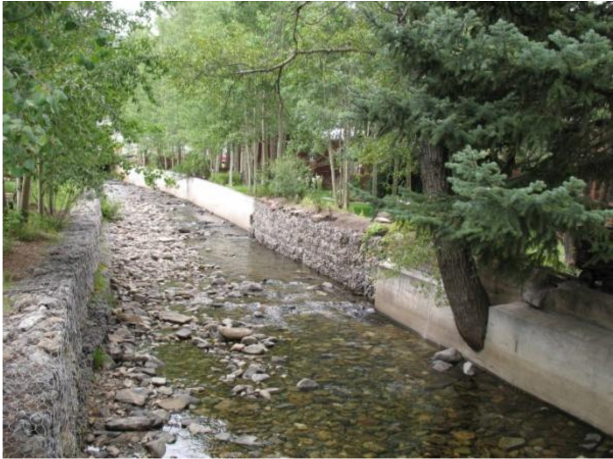
Photograph 3. Photograph taken August 2009 looking upstream along Coal Creek in the Town of Crested Butte from the Totem Pole Park bridge. Note the channelization of the creek with gabions and concrete and the resulting reduced riparian zone.
