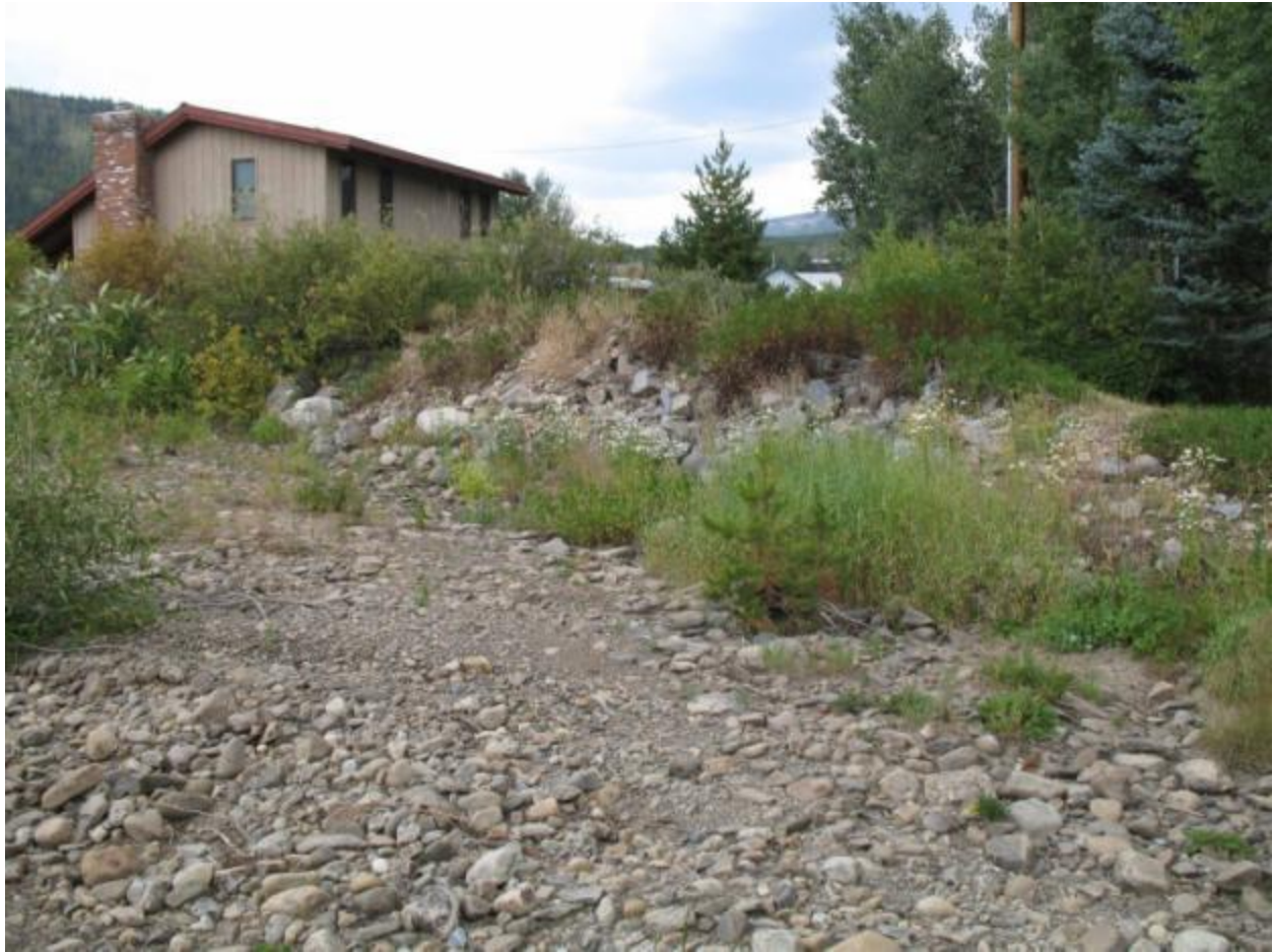
Photograph 6. Photograph taken August 2009 looking across Coal Creek in the Town of Crested Butte near Third Avenue. Note the channelization of the creek, berming to reduce flooding and the disturbance from diversion maintenance.
