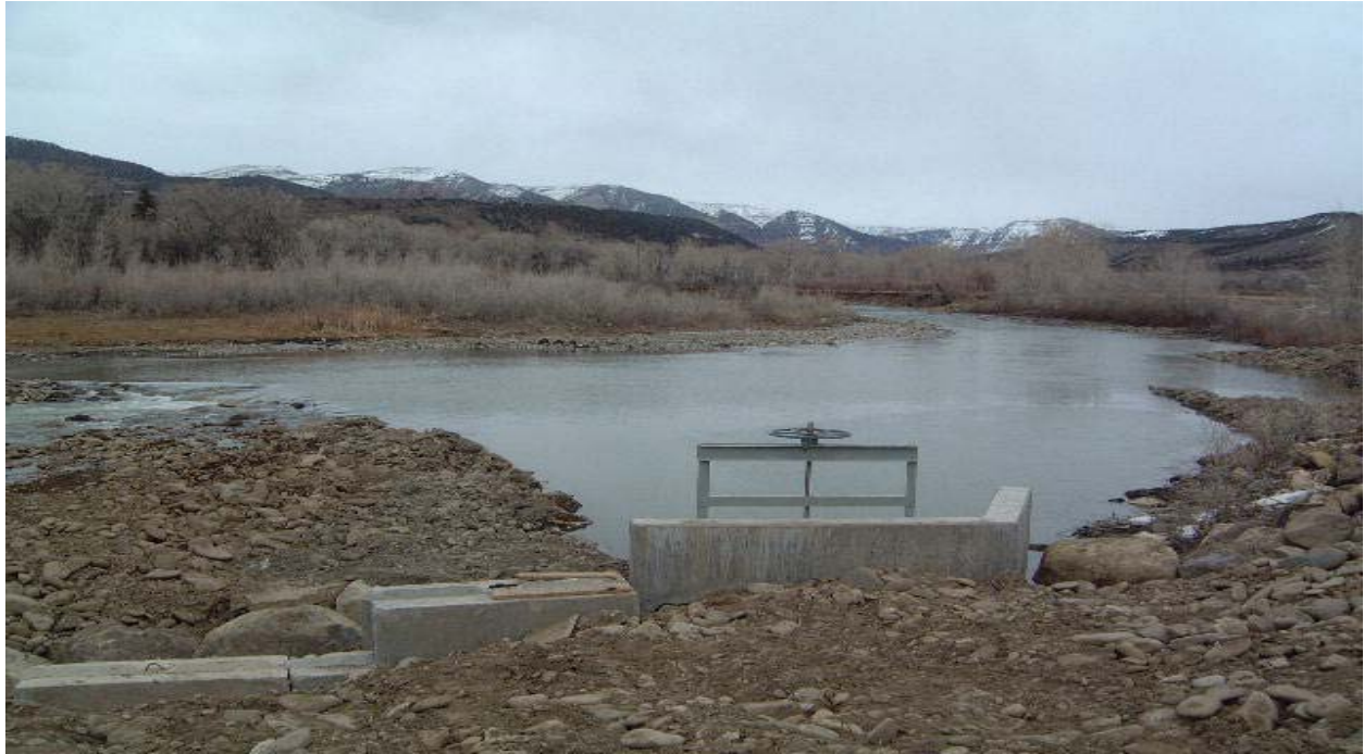
Photo 3. Completed low-flow channel and energy-dissipating plunge pools below diversion, view upstream. 2008.
