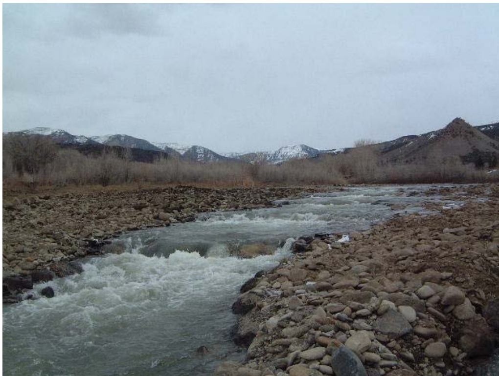
Photo 3. Completed low-flow channel and energy-dissipating plunge pools below diversion, view upstream. 2008.
