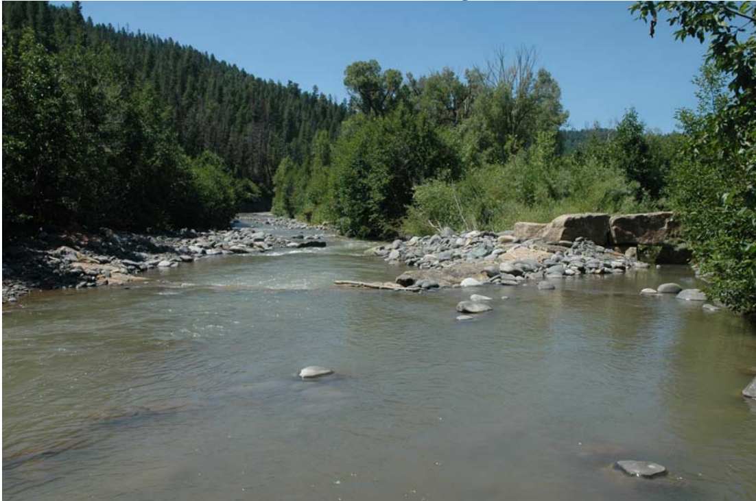
AFTER: Rock diversion controlling flood water into side channel, channel narrowing and induced meandering downstream
