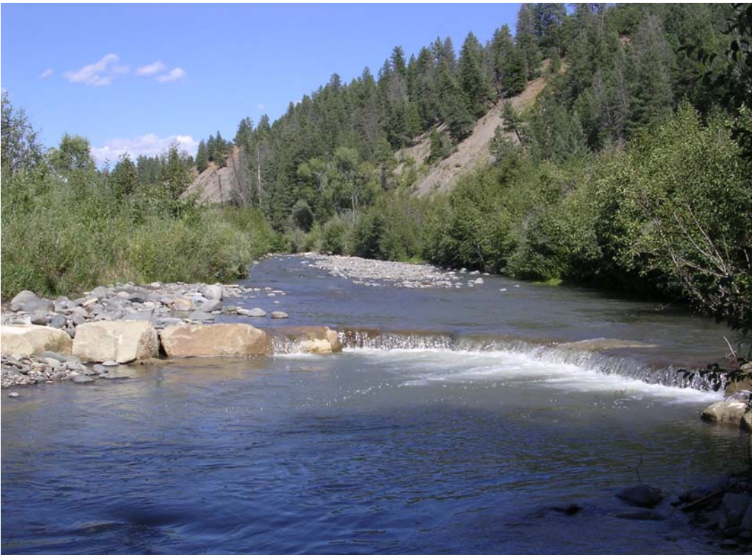
AFTER: Constructed channel bar to promote deeper narrower channel with cross vane for habitat and bank stability.
