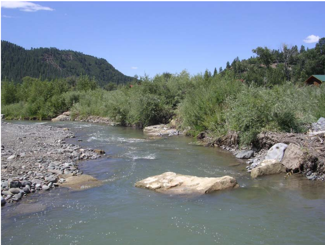
AFTER: Single channel with rock bank protection and habitat rock
