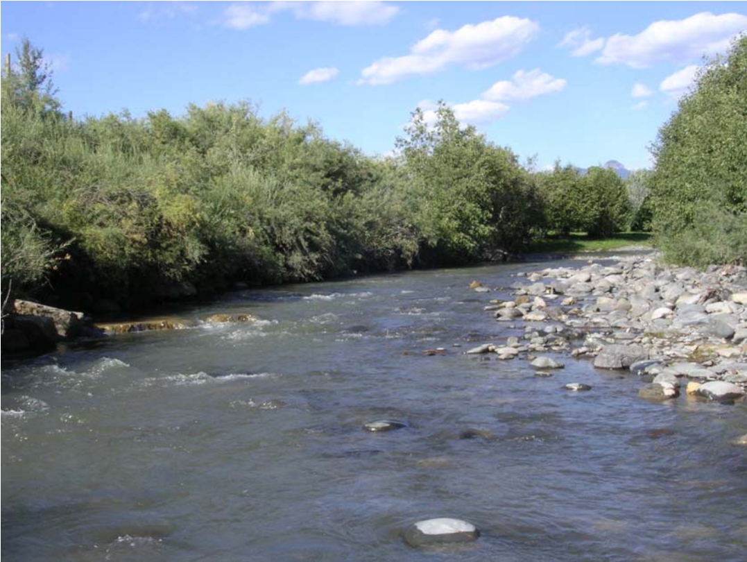
AFTER: Enhanced point bar to promote deeper narrower channel with short rock vane for habitat and increased bank stability.
