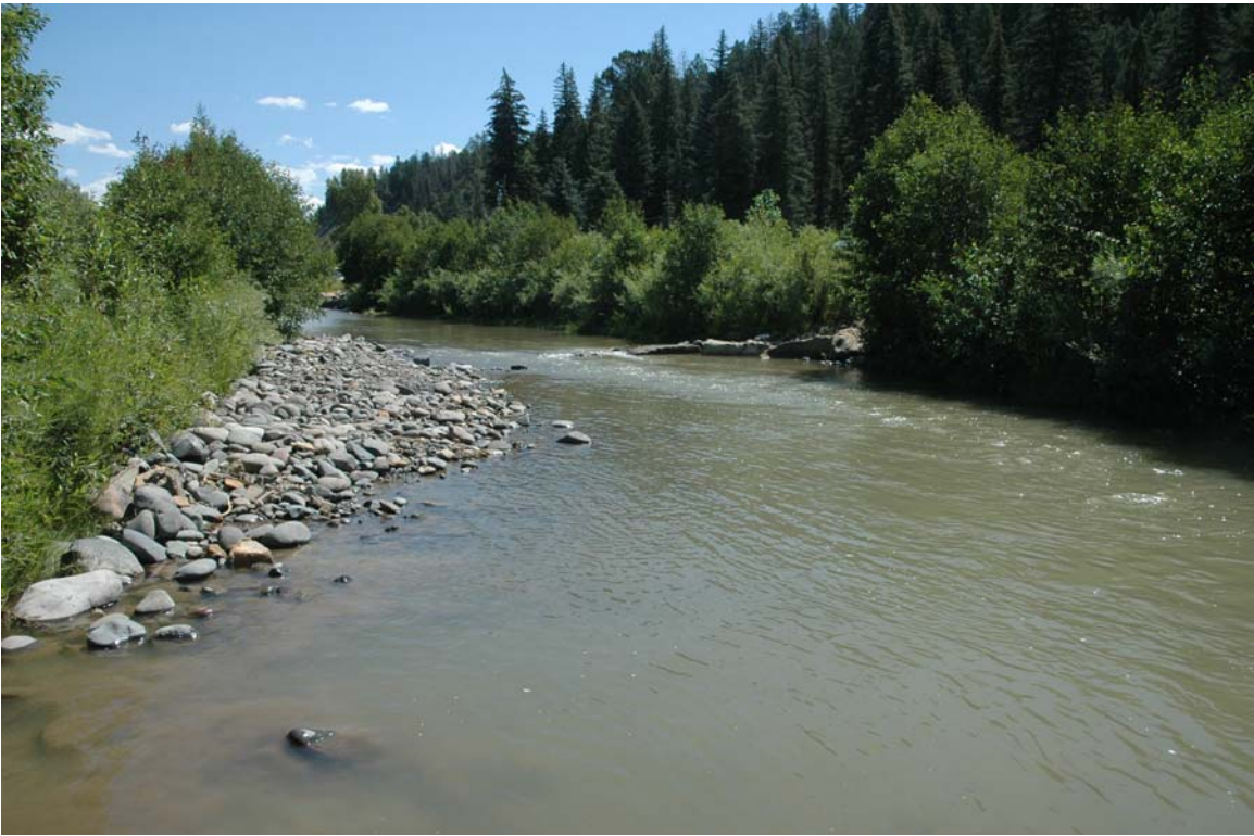
Photo 2. Photo of newly constructed alternating bar with dense bank vegetation. Note the rock structure and deeper water river-left, creating good fish holding potential beneath the overhanging Alder bushes.
