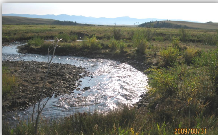
Figure 3: A new bench was created on this rapidly eroding bank during phase 2. The bench was planted with willows and wetland sod, and the channel was realigned to decrease near-bank stress. The bank will eventually continue to erode, but at a slower natural rate now that the appropriate vegetation will be in place.
