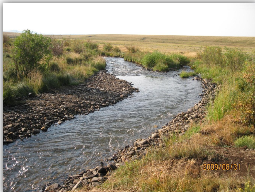
Figure 2: Channel shaping and bank toe treatments were completed in phase 2. The bank toes are constructed of streambed gravel and cobble that can be moved by the stream within a few seasons of high flow. They serve as protection for the banks while planted sod and willows take hold. The channel was gently reshaped to enhance the thalweg, to make the channel deeper and narrower at low flow, and to create pool area. Only native bed materials were used, so the channel is still free to readjust and adapt naturally.
