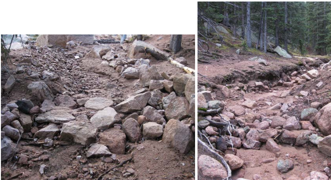
Figure 3 and 4. Completed Cross-vanes in Lower Sub-Reach of Ski Creek.
