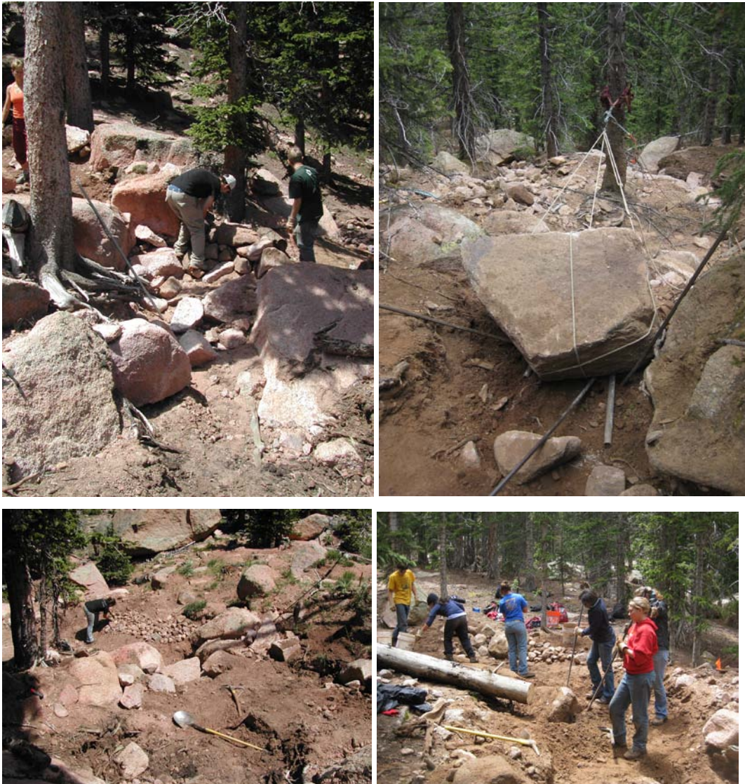
Figure 5-8. Pikes Peak Corps crew completing bank stabilization.
