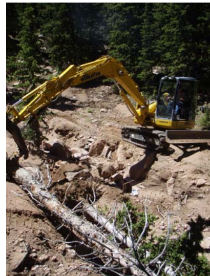
Figure 1. Installing bank stabilization structure
