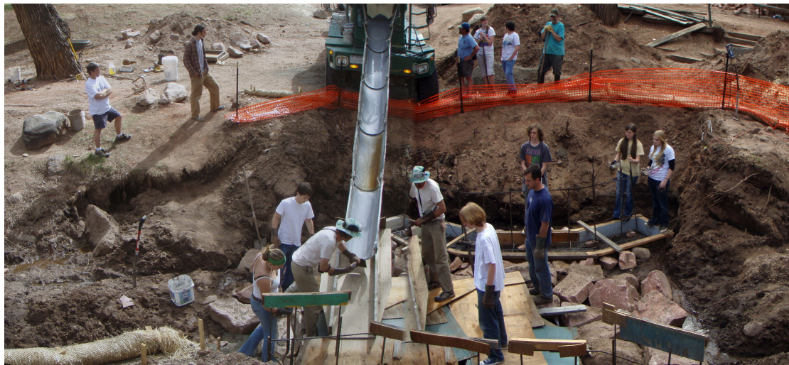
Manitou Springs HS Students pouring bridge footings under the direction of CC staff.
