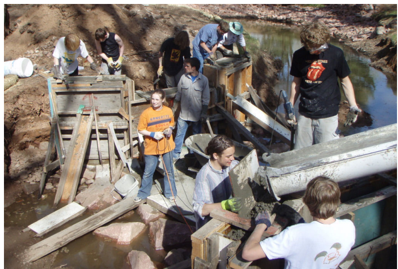
Pouring the Bridge Foundation Wing Walls.
