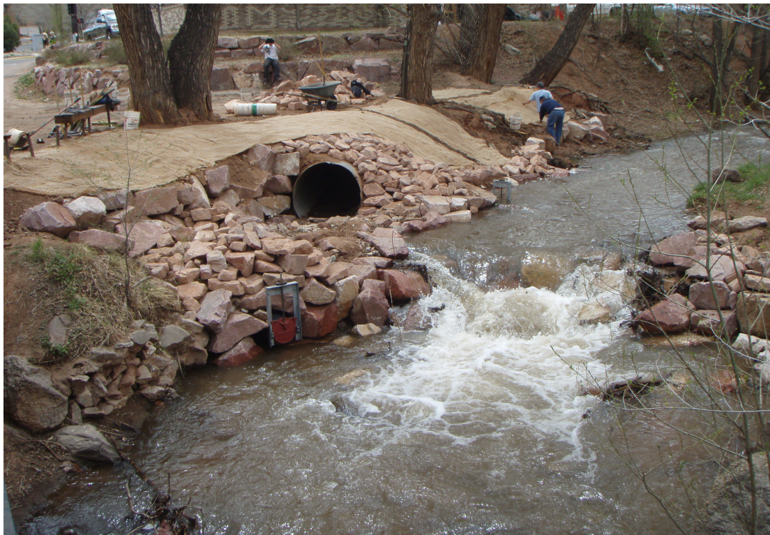
Post-project pond Dual Head-gate diversion structure with 48" storm water culvert.
