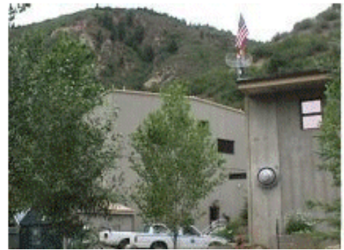
Red Mountain Water Treatment Plant
