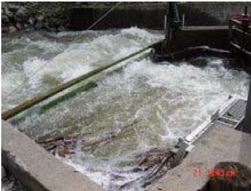
Figure 5: No Name diversion structure
