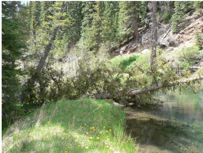
Photo 7.6. The Breach along the Rico Boy/Santa Cruz Settling Pond Created by a Fallen Tree.
