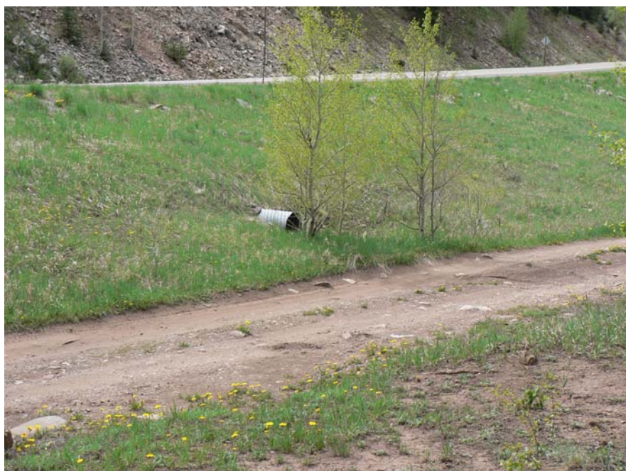
Photo 7.1. Example of Stormwater Impacts created by Recreator Activity. (storm drain located on top of a dirt road accessing an unrestricted campground adjacent to the Dolores River).
