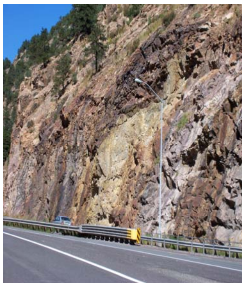
Road cuts through the sulfide ore body leaving behind actively eroding rock faces.
