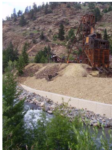
New retaining wall at the Maude Munroe to keep flood waters out of the mill waste pile.
