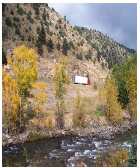
I-70 road bed built on mill tailings containing hazardous metals including mercury, cyanide, cadmium, zinc, and arsenic.
