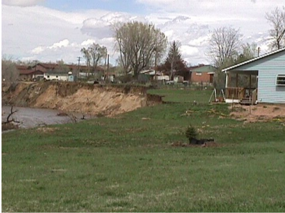
Photo 4-22: Streambank erosion encroaching on homes on the banks of Fountain Creek in the City of Fountain.
