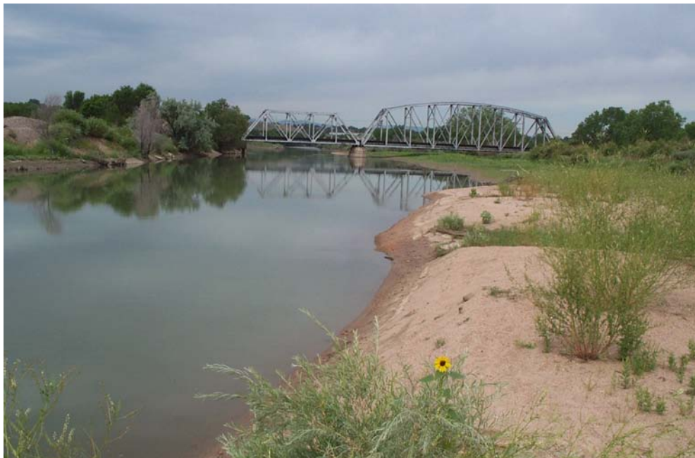
Photo 4-25: View looking upstream on the Arkansas River showing sediment prograding into the river from Fountain Creek and the pool formed in the river due to flow constriction at this point.
