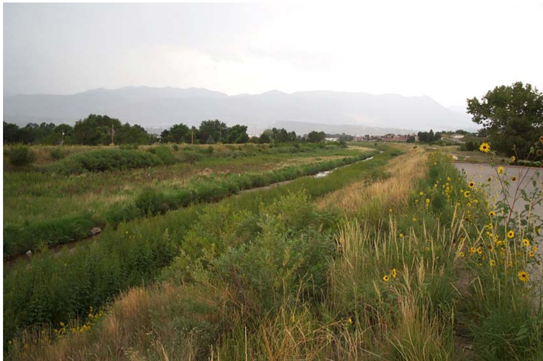
Photo 4-19: The Templeton Gap Floodway diverts storm runoff from the upper Shooks Run drainage to Monument Creek to relieve flooding problems.
