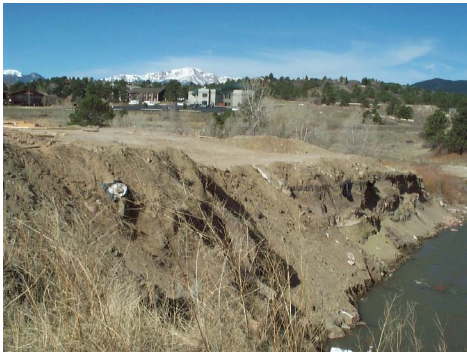
Photo 4-9: Fill placement in the Monument Creek floodplain at a new motel development in north Colorado Springs restricts channel flow capacity.
