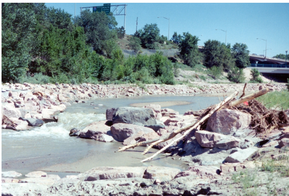
Photo 4-15: One of the boulder drop structures recently constructed on lower Monument Creek in Colorado Springs.
