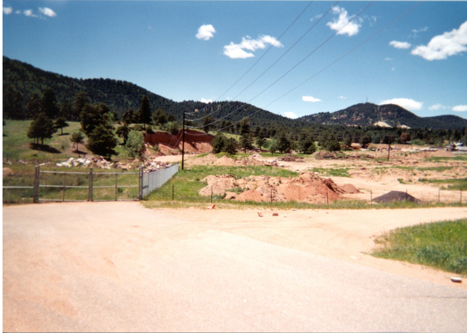
Photo 4-2: Realignment of upper Fountain Creek channel has pushed the channel to the southwest side of the valley, causing bank erosion downstream of Woodland Park.
