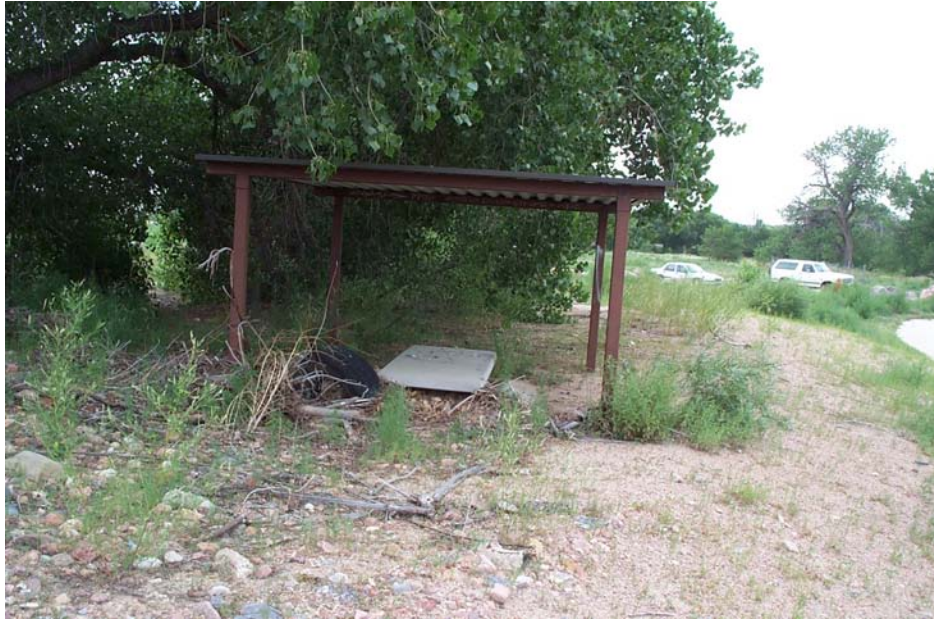
Photo 4-26: Several feet of sediment covered the park area near the mouth of Fountain Creek during the 1999 flood as is shown by this picnic table, the top of which now appears to be only a few inches off the ground surface.
