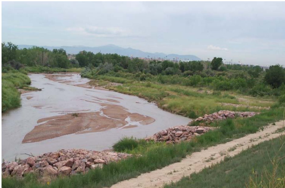
Photo 4-31: Severe bank erosion was a problem at this site near the Creek Side Subdivision in north Pueblo. Spur dikes have been constructed at this location to control erosion in the future.
