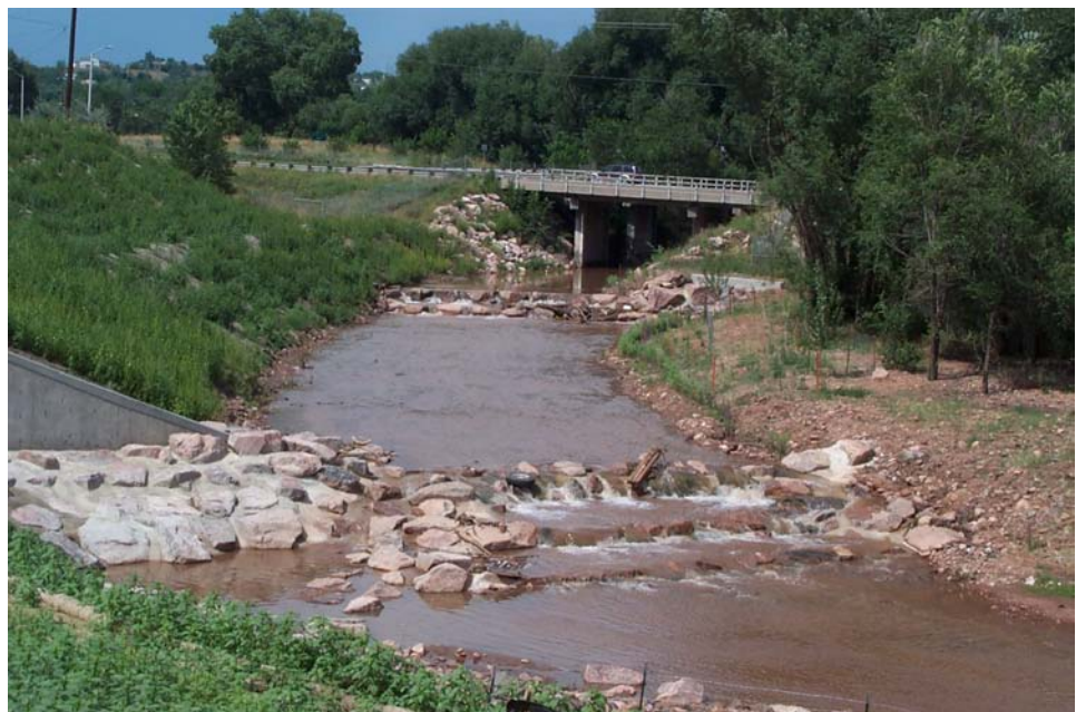
Photo 4-6: Fountain Creek improvements near 21 st Street.
