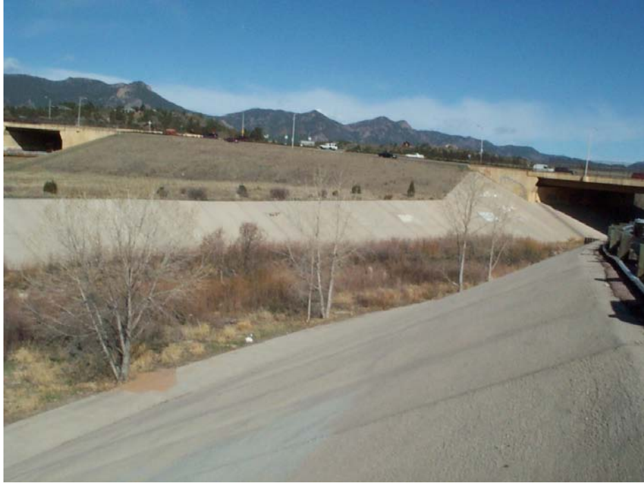
Photo 4-10: Concrete channel lining at the Woodmen Road Bridge provides bank protection and restricts the floodplain width.
