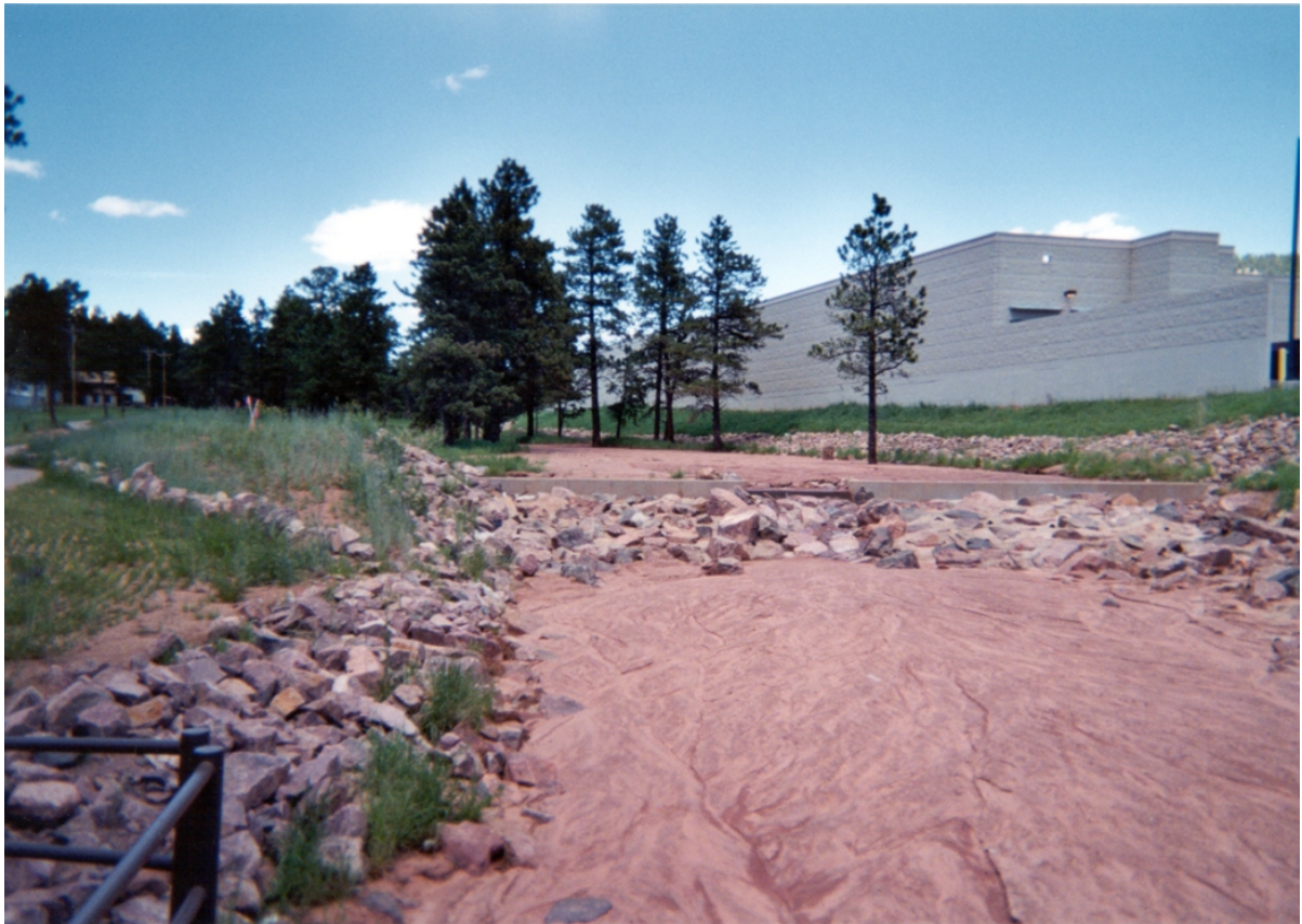
Photo 4-1: Sediment in the upper Fountain Creek channel in Woodland Park.
