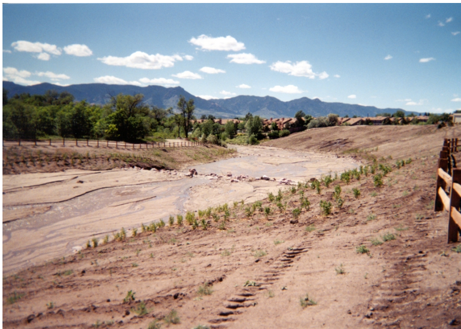
Photo 4-14: A new boulder drop structure to control channel degradation on Cottonwood Creek downstream of Union Boulevard.
