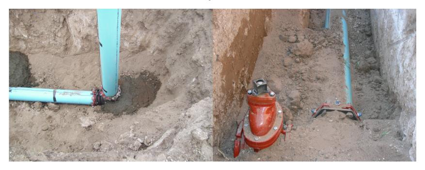
This is a concrete Thrust Block at 90-degree elbow that will go into the Water Treatment Building.
