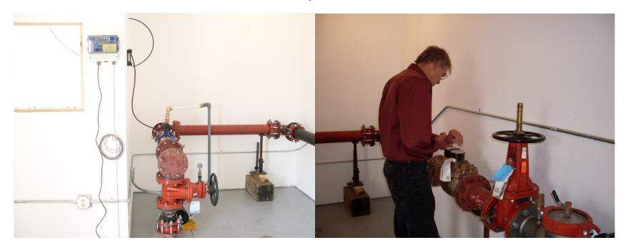
The Chlorine Injection system is located in the window to the left and feeds through the wall into the system.
