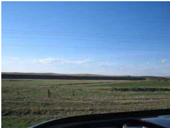
Looking west at Ramah State Wildlife Area Dam
