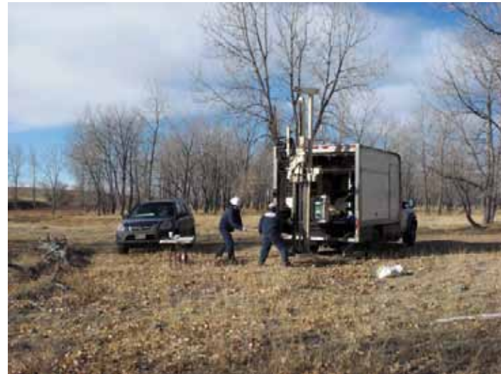
Geoprobe Rig at GP28 location east of Simla
