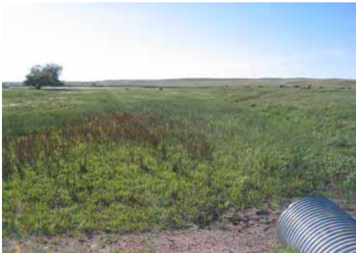
Stock pond discharge pipe and small phreatophytes near Matheson
