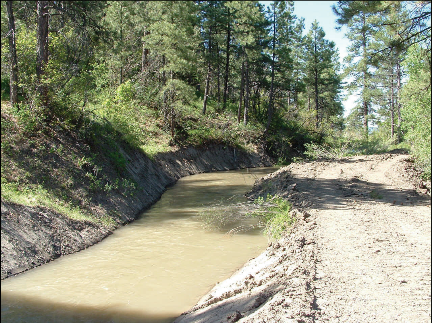
Park Ditch after temporary repairs. The proposed pipe will be placed in the exposed undisturbed shale on left of photo.
