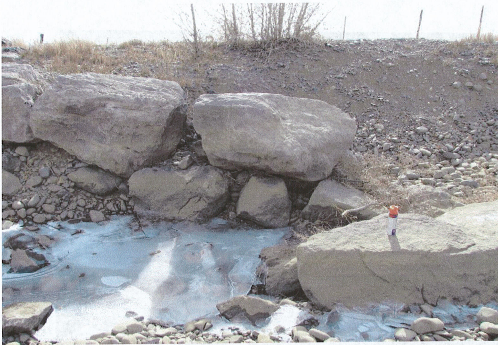
Figure 10: Lack of footers and gaps between rocks caused this failure.
