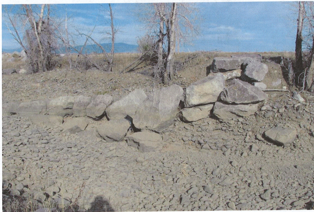
Figure 7: Failed Structure. Lack of proper footers.
