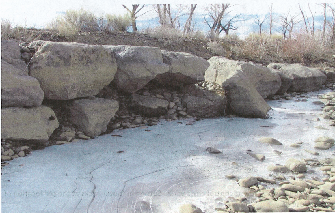
Figure 5: Failed Vane Structure
