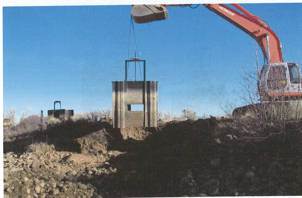
Figure 15: Re-setting the San Jose #1 head gate
