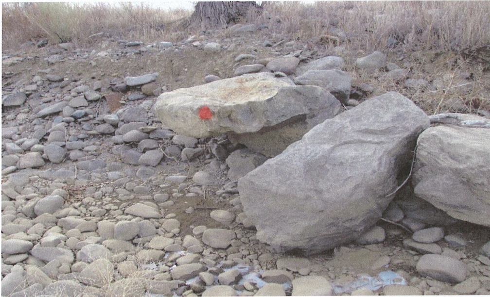
Figure 8: Failed Structure. Lack of footers.
