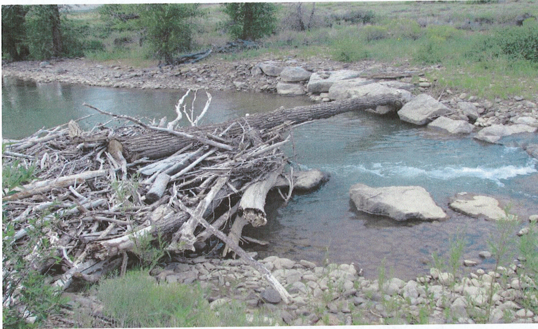
Figure 12: Rivera Irrigation Diversion. Lack of footers and gaps in-between rocks combined with the entire structure built narrow. Great fish habitat but poor irrigation diversion.
