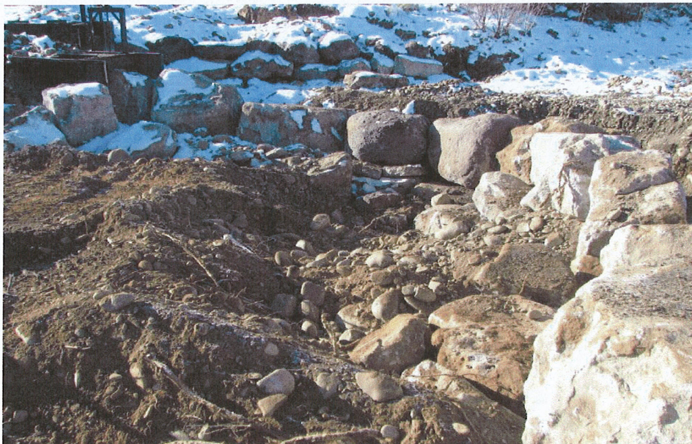
Figure 19: Completed Cross Vane on San Jose #1 prior to backfilling
