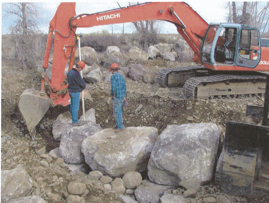
Figure 18: Steve Belz instructs Randy of proper installation of cross vane structure.
