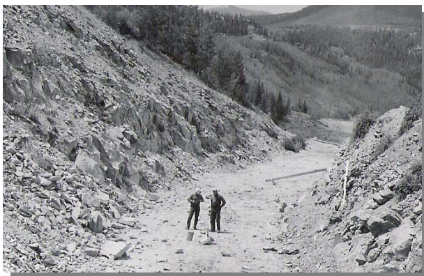
The emergency spillway in 1958 (Photo courtesy San Luis Valley Irrigation District).
