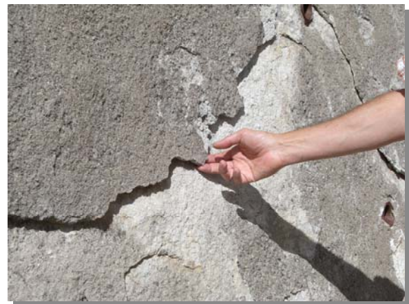
Concrete spalling and cracking in the spillway chute
